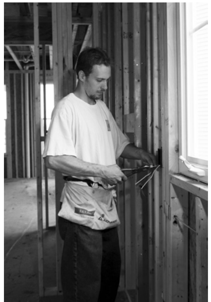
An electrician prepares the wiring for an interior room.
