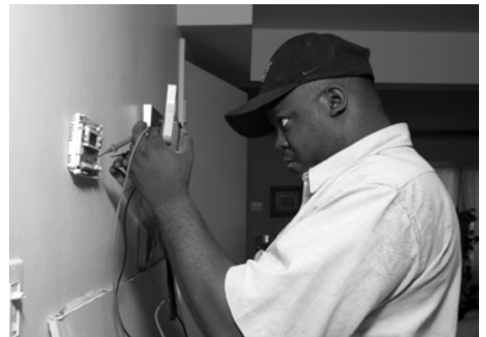
A heating, air-conditioning, and refrigeration mechanic works on a thermostat for a heating and air-conditioning system.
